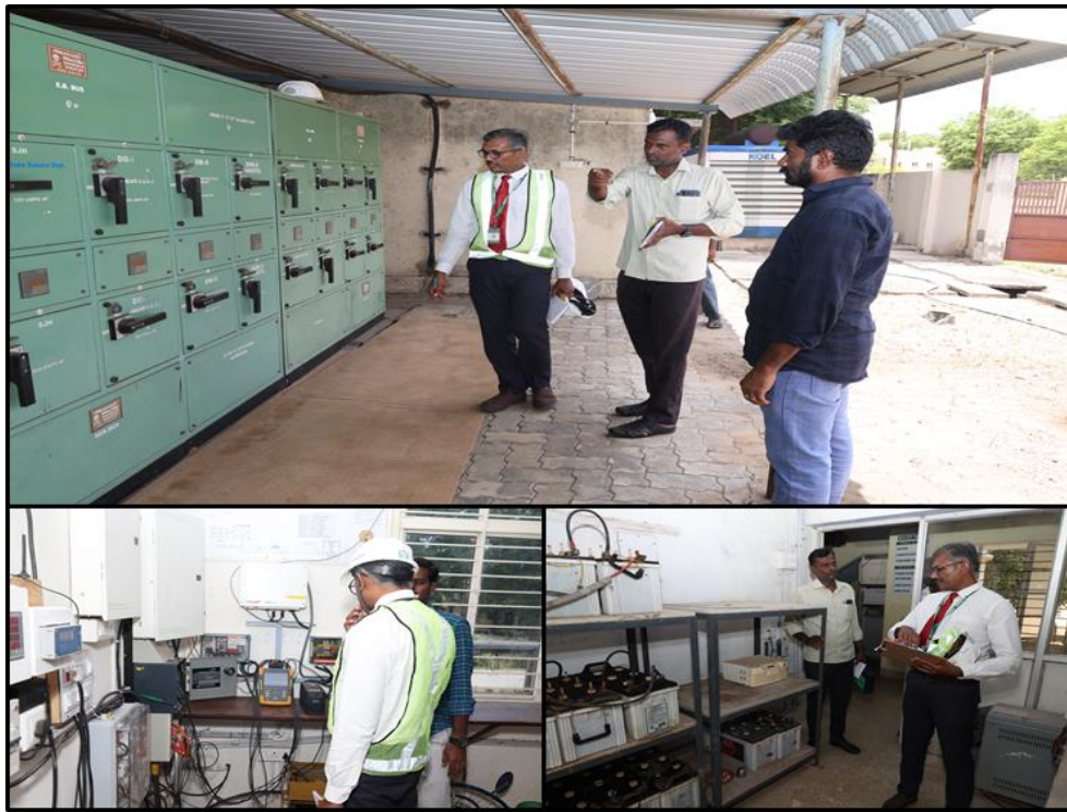
Energy conservation facilities observed in the Campus
